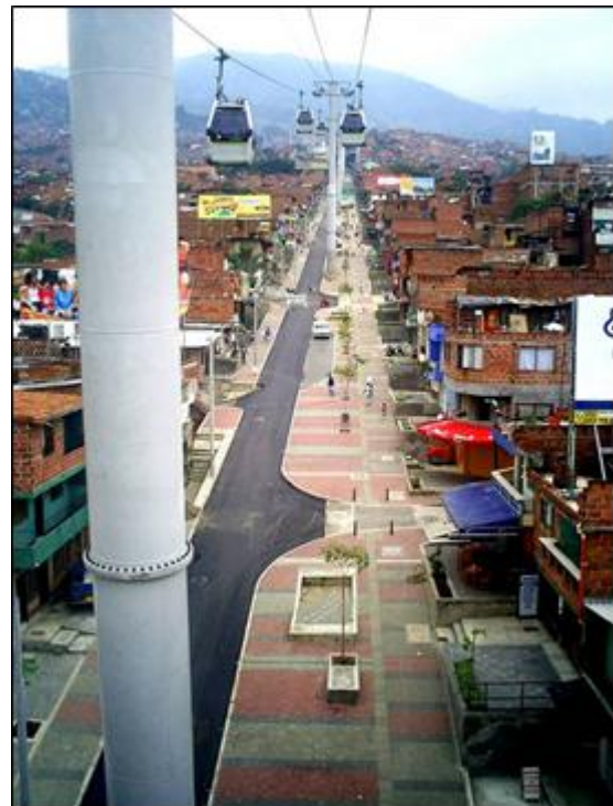
PHOTO 5. METROCABLE LINEA K ACEVEDO - SANTO DOMINGO
