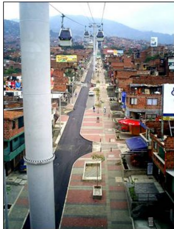
PHOTO 5. METROCABLE LINEA K ACEVEDO - SANTO DOMINGO
