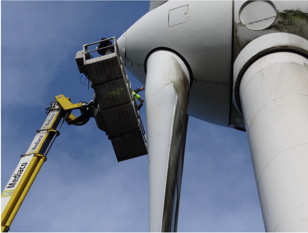
Figure 4.10: Aerial work platform positioning
