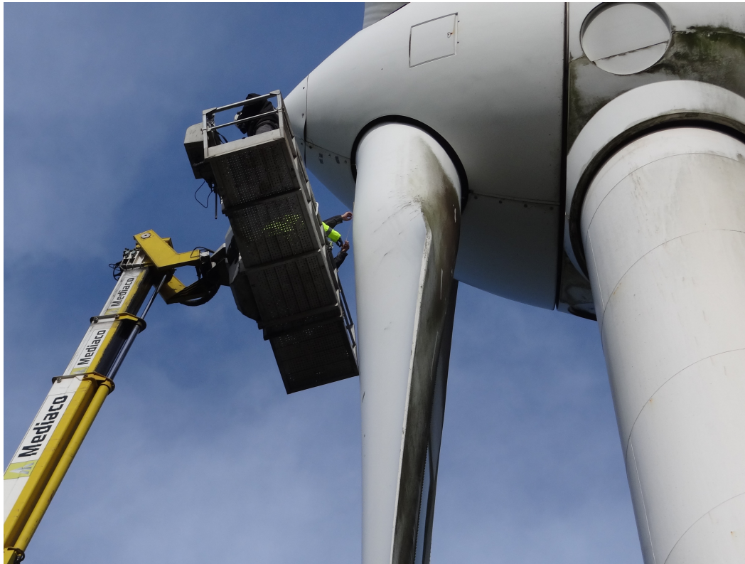
Figure 4.10: Aerial work platform positioning
