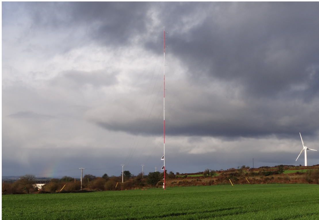
Figure 4.8: Photo of the met mast after its installation
