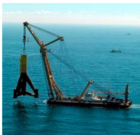
Figure 1.27 – Structure tripode
