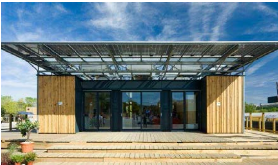
Figure i.16 – Sumbiosi house at the Solar Decathlon Europe 2012.
