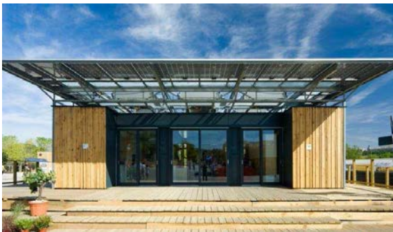
Figure i.16 – Sumbiosi house at the Solar Decathlon Europe 2012.
