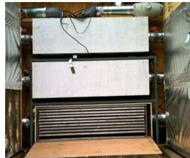
Figure i.19 – PCM system embedded in the Sumbiosi house wall at the IUT campus in Bordeaux.
