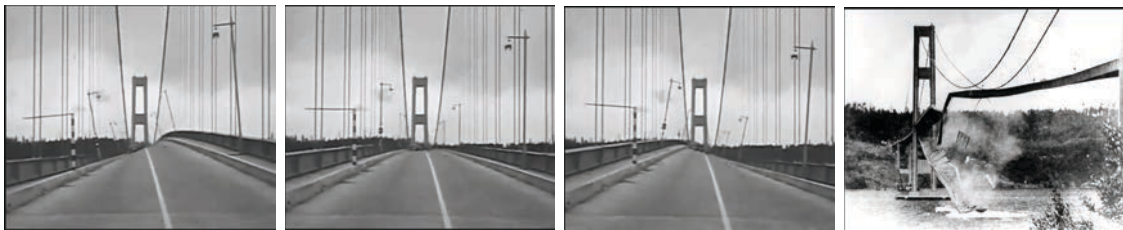
Figure 1.1: Tacoma Bridge Collapse - November 7th, 1940
