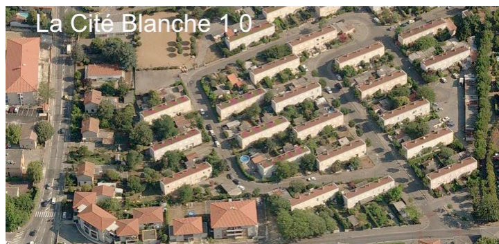
The Cité Blanche before refurbishment (1)
