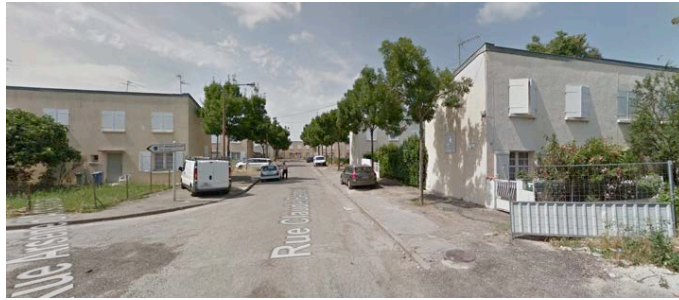
The Cité Blanche before refurbishment (2)
