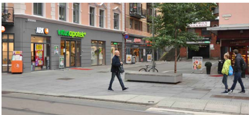
Though entrance to a parking garage, the sidewalk is continued, which eliminates barriers such as edges, etc. The bench offer a possibility to sit down, with weather-protection from the tree (as it gets bigger).
