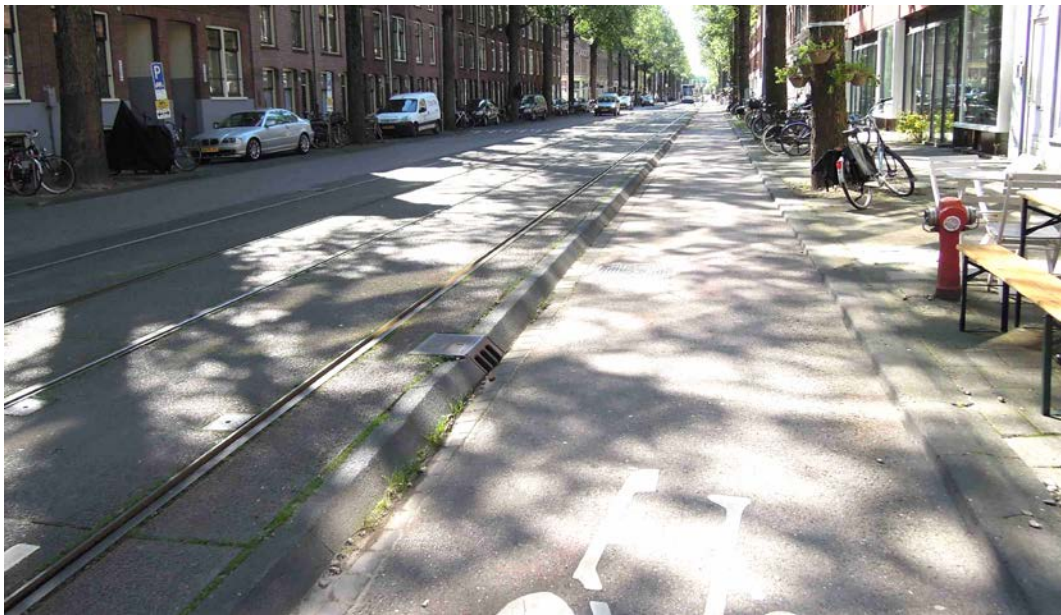
Cycling infrastructure separated from the sidewalk and the car/tram lane by physical barriers, Amsterdam (Netherlands)
