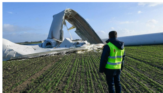
Figure 0.1: Collapsed wind turbine in Bouin, France. It is attributed to extreme winds that occurred during the Carmen storm that hit western France in early January 2018. The turbine had been in place for 15 years. It is worth noting that it resisted several similar and even stronger storms, such as Xynthia in February 2010.
