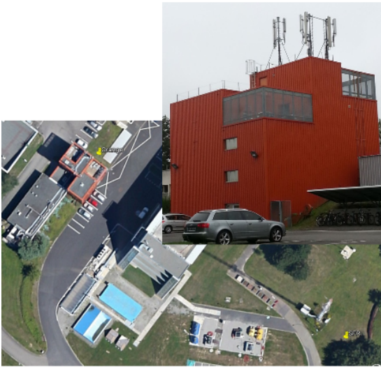
FIGURE 2.10 – Station de base Orange
