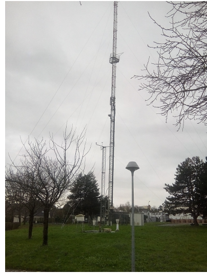
FIGURE 2.11 – Station de base SFR
