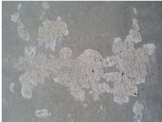
FIGURE C.5 – L'écaillage (Shea, 2018)
