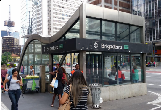
(a) Subway station entrance
