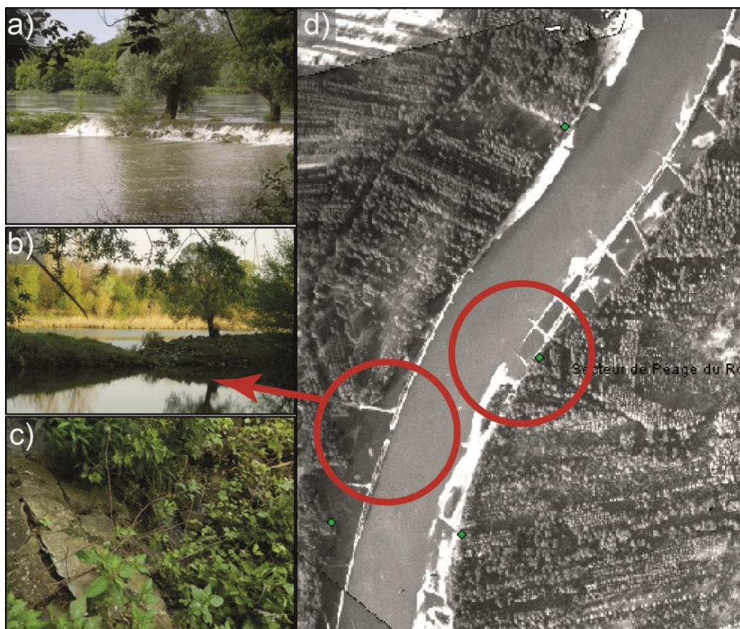
Figure IV–8: Dike fields are connected to the main by-passed channel by various mechanisms: a) submersion, b) passages, c) ‘seepage’. Aerial image source: IGN©.
