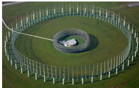
Figure 2.18: Wullenweber antenna next to Augusta in Germania
