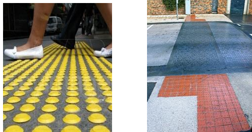
Figure 3.3 Surface of the path specially made for VIP
