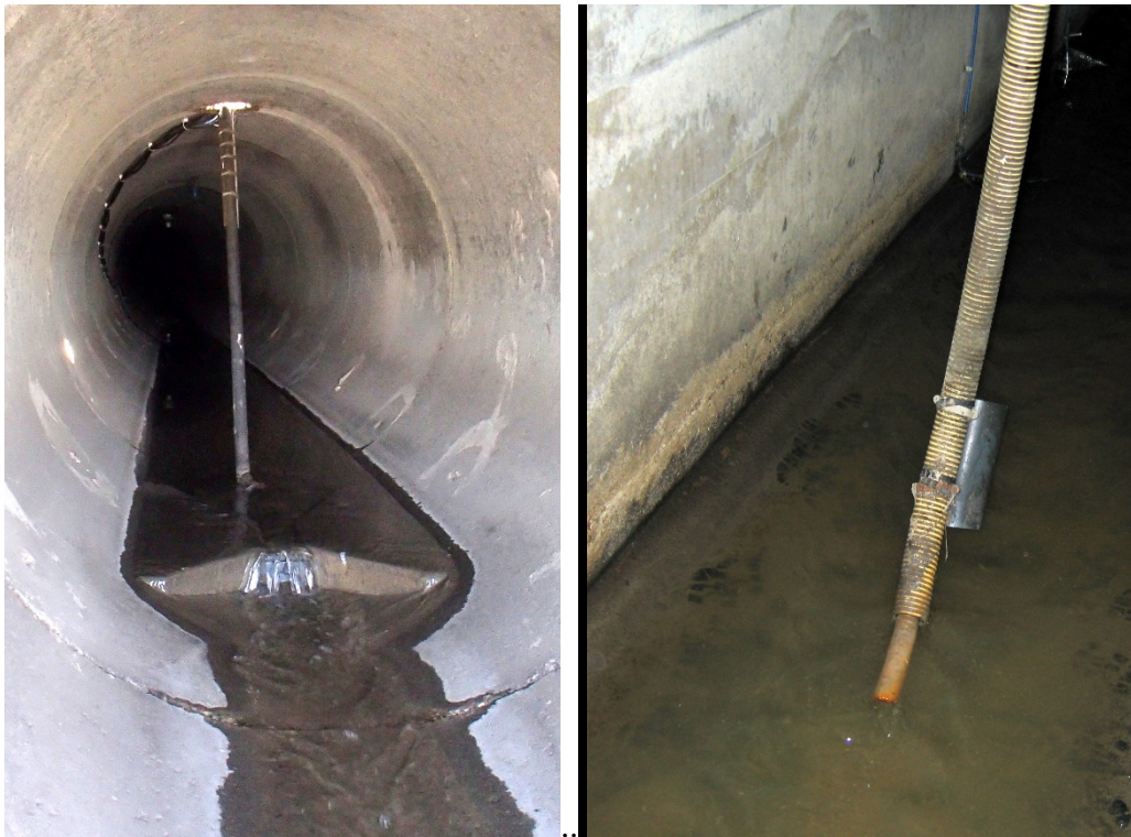
Figure 12. Sampling tube in the Chassieu sewer. Left: general view with the sampling tube located just upstream a Venturi flume created to ensure a minimum water level for sampling; Right: detail of the lower part of the sampling tube immersed in the flow.
