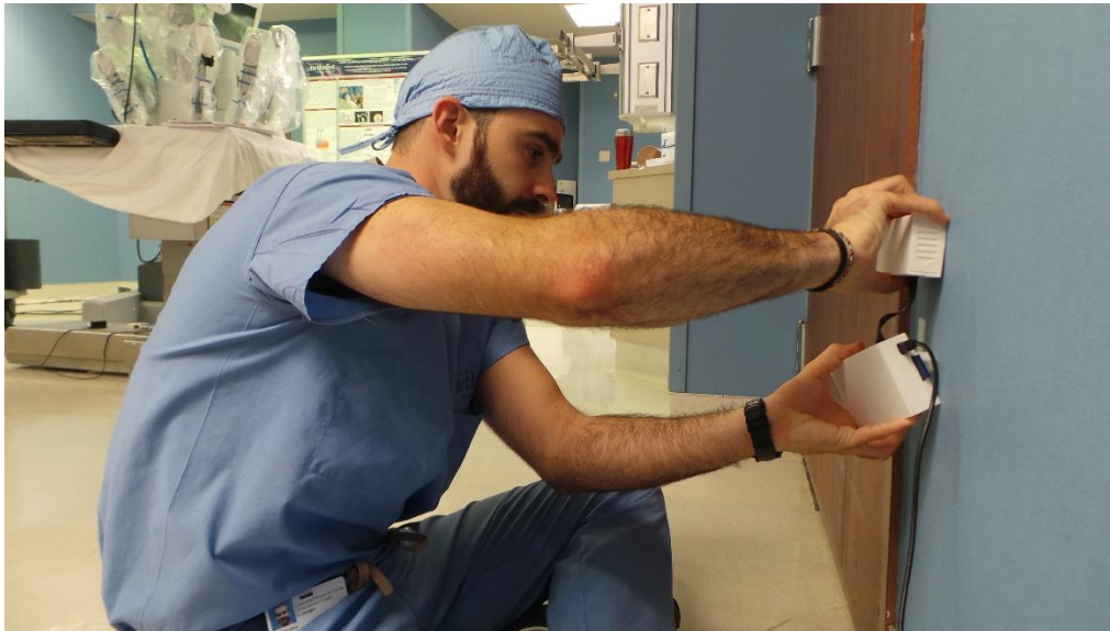
Figure 22. A colleague installing a SmartOR door sensor for detecting opening and closing.
