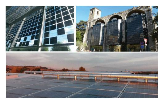
Fig. 1.6 BIPV systems, (top left), integrated solar cells on the outer skin of a double skin façade at the Schneider electric building, Grenoble, France, (top right), similar system at the tourism office of Alès, Cévennes, France, (bottom) assisted hybrid thermal-photovoltaic designed with EPC Solaire in the context of the ADEME project Horizon PV
