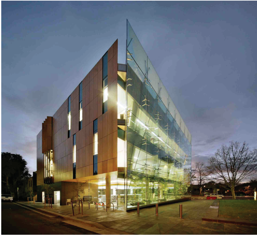
Fig. 1.5 Vegetalized double-skin façade on the Surry Hills Library and Community center, Surry Hills, Australia Credit: Prodema
