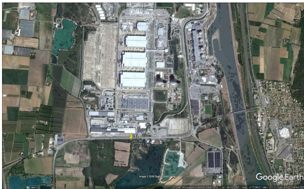
(a) (1) - Power plant
