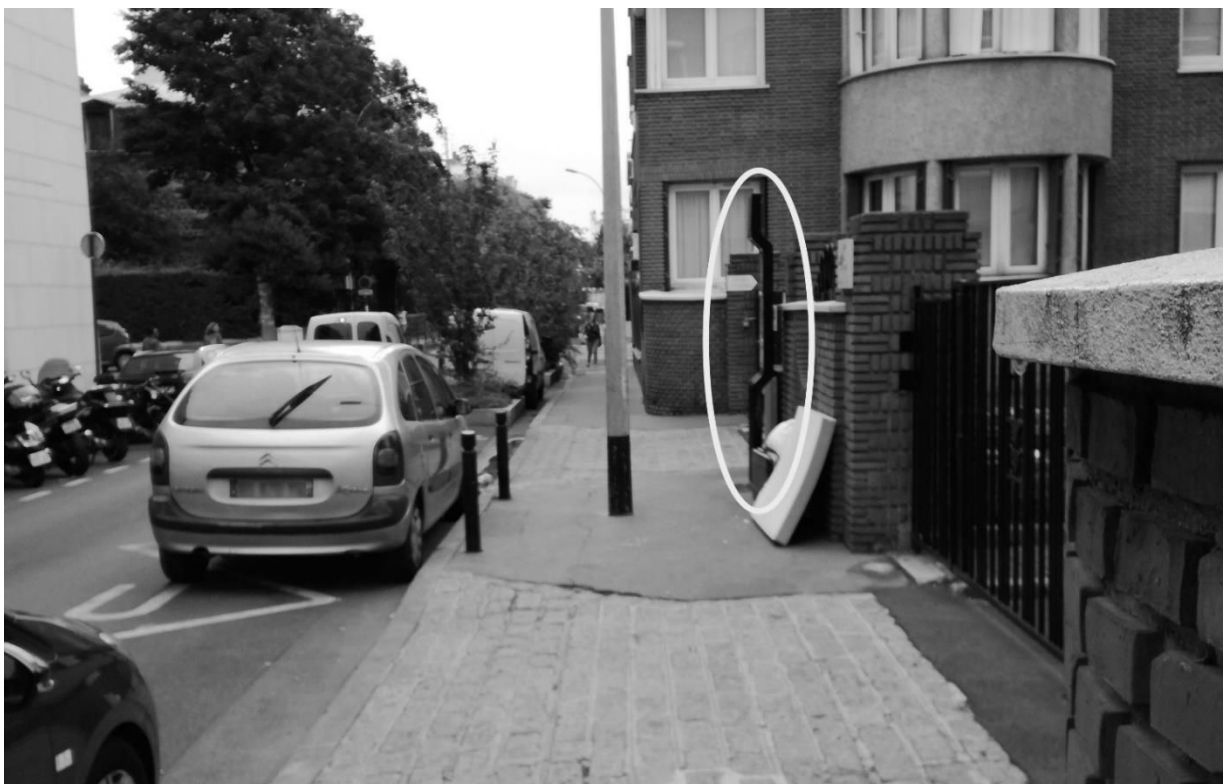
Figure 33. Barely visible bus stop
