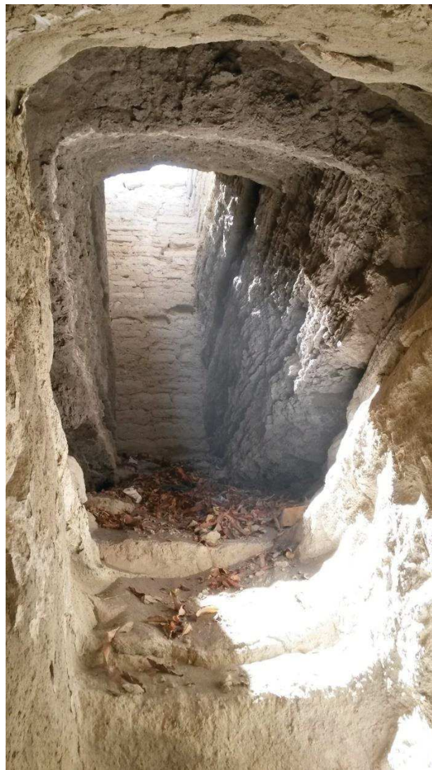
Figure 22 : Typical shaft well (Lumbrera) in Pica area
