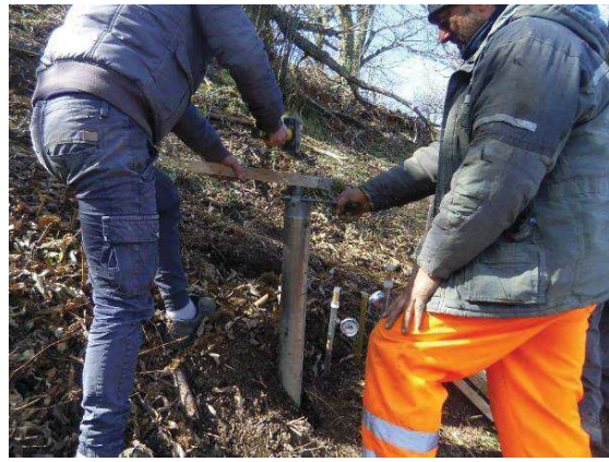
Figure 97 – The tube is being pushed into the soil using a hammer.
