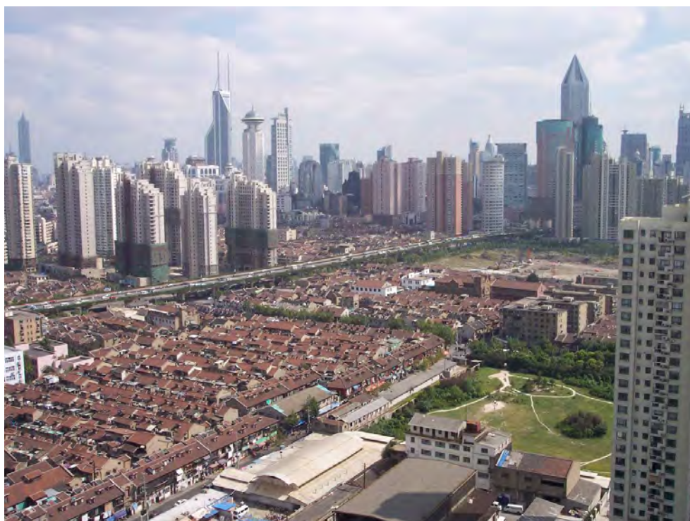
Figure 0-30 Aerial view of Shanghai, 2004. Renee Y. Chow, «In a Field of Party Walls, Drawing Shanghai's Lilong», Journal of the Society of Architectural Historians , Vol. 73 No. 1, March 2014, pp. 16-27.
