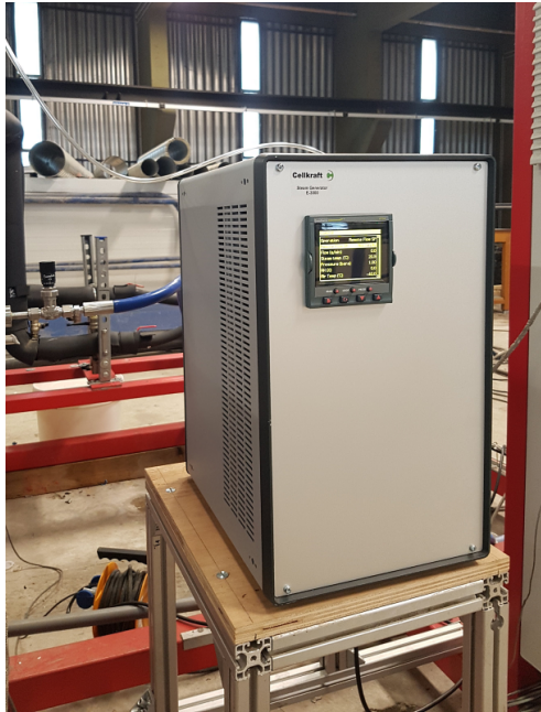
Figure 2.12 – Precise steam generator unit for the air handling unit
