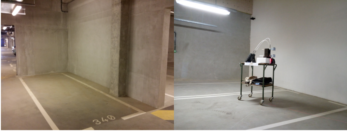
Figure 5.26 – Wall and measurement setup.
