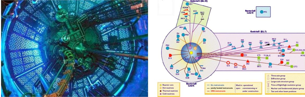
Figure 2.5: **Picture of the high-flux reactor Institut Laue-Langevin (ILL).** Left: view of the pool where the core of the reactor is contained. Right: Distribution of the different kinds of neutrons to the instruments.
