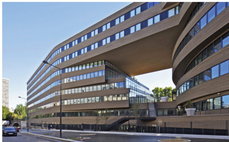
Figure 1.5 – Pushed Slab Building 1-11 rue Brillat Savarin, 75013, Paris
