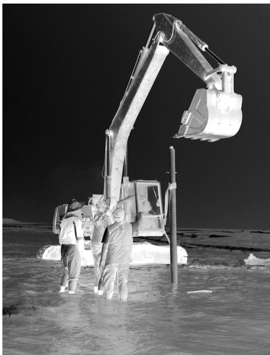
Figure 3. Instrumentation deployment. Pressure data loggers are protected inside 6m long steel tubes and sensors plugs pass through the tube wall.
