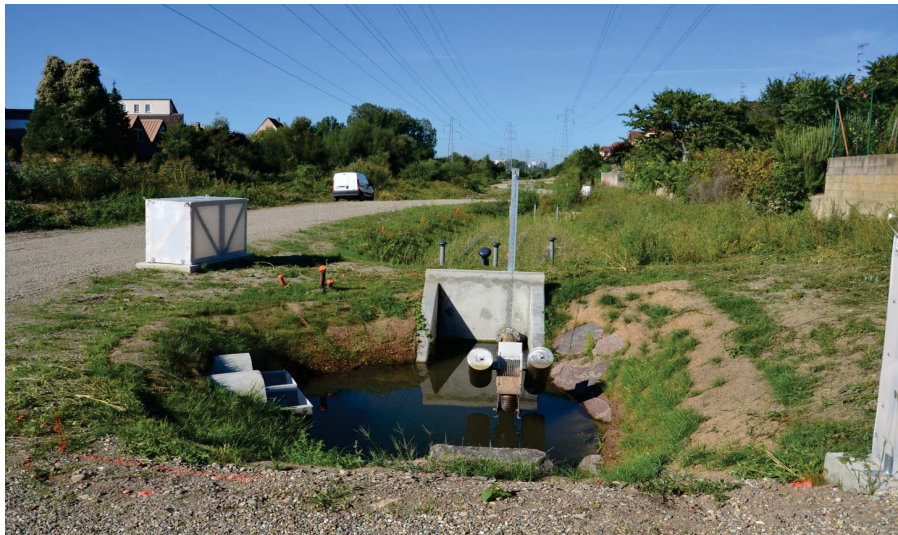
Figure 5.5: Ostwaldergraben site, the sedimentation pond (front) and the constructed wetland (behind)
