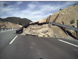
Fig. 7.7a-b. Major slip-off of the Diezma Landslide on the  $18^{th}$  of March 2001 (photos by courtesy of: JUNTA DE ANDALUCÍA, CONSEJERÍA DE OBRAS PÚBLICAS).
