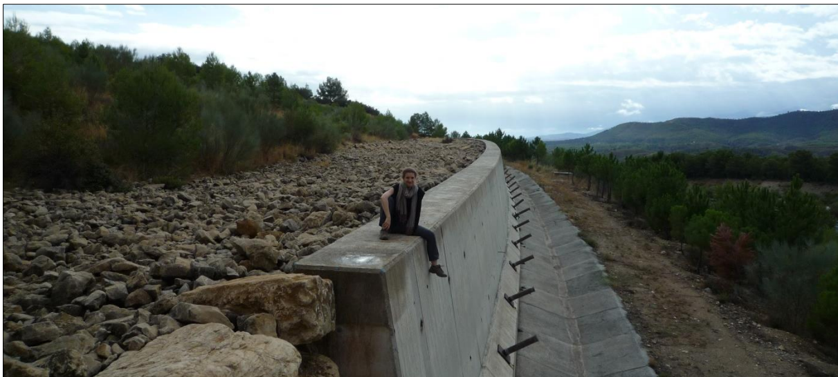
Retention wall of the Diezma Landslide (9 th of September 2018).
