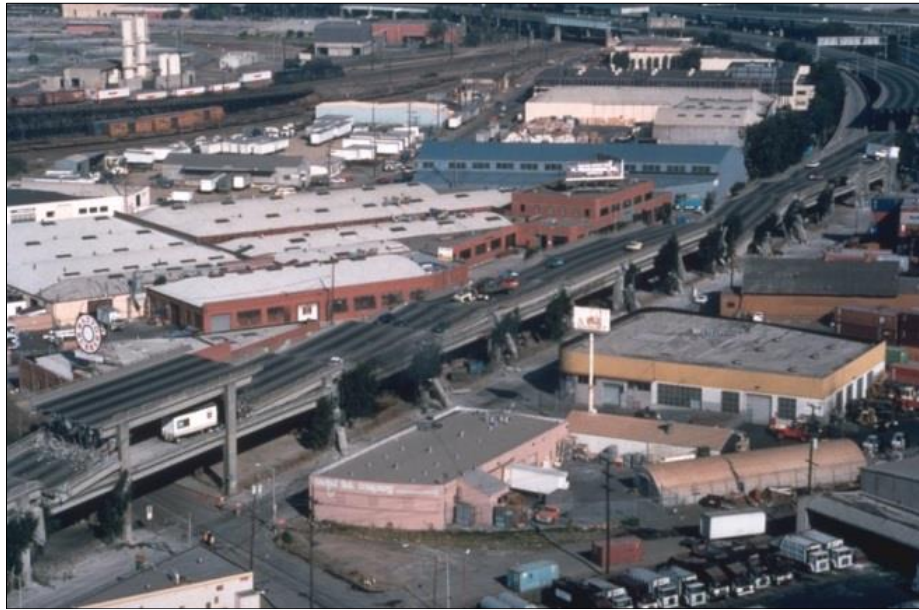
Fig. 1.4. Collapsed Cypress Viaduct in Oakland (LEWIS, 1989).
