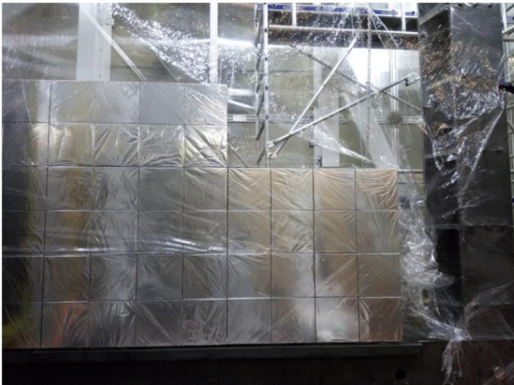
Figure 3.20: Front view of one main wall during its assembly at LSM. The wall is built by assembling the bricks (8 by 8).
