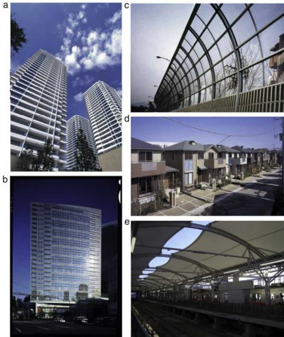
Figure 2.14. Application of self-cleaning building materials for a) self-cleaning tiles, b) self-cleaning glasses, c) self-cleaning sound proof wall on a highway, d) self-cleaning of tiles and glasses, and e) self-cleaning roof of a train station. Reproduced from ref 72 .
