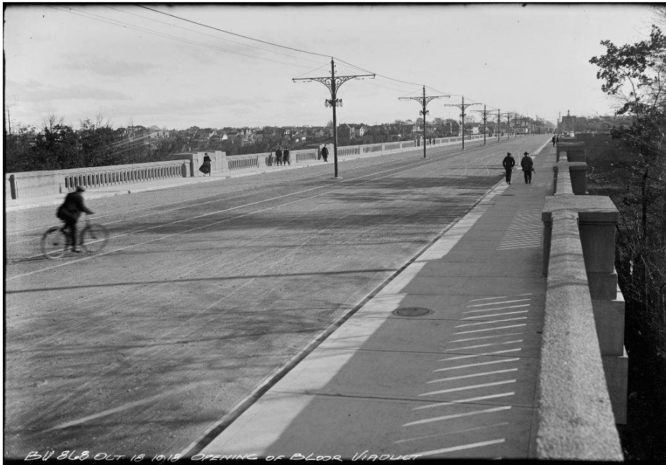
Figure 4 : Arthur S. Goss, Traffic, Bloor St. Viaduct
