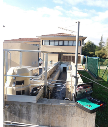
WWTP of La Crau
