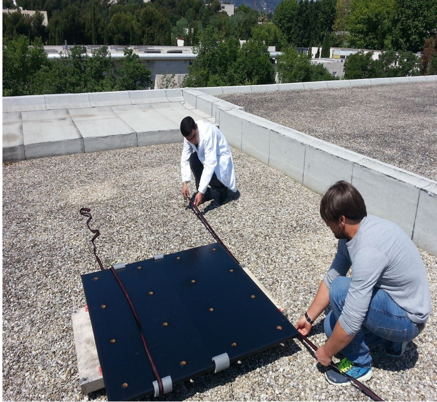
Figure II.8: Image showing the installation of the wooden plank on the roof of the MIO laboratory (Ex-Protée) ( 43^{\circ} 08' 11.2'' N 6^{\circ} 01' 16.7'' E).
