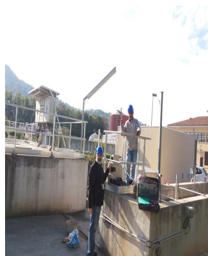
(b): WWTP of La Crau City
