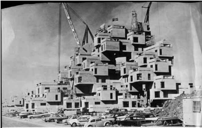
HABITAT 67 BY MOSHE SAFDIE DAVID, BAROTT, BOULVA ASSOCIATED ARCHITECTS
