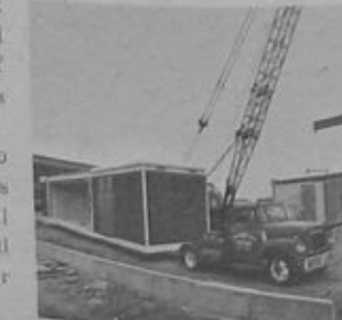
Illustrations (from top down) show typical Habitat box raised into position by special crane; "hushair" vacation cottage and metal shipping container being airlifted by helicopter; diagrammatic model of Le Corbusier's Marseilles apartment as envisaged by him in 1946; prefabricated, Soviet apartment unit of concrete hoisted into place—after having been trucked through Moscow streets; and the standard Mobile Home unit used in the construction of Syntex offices (p. 46), being trucked to building site.
