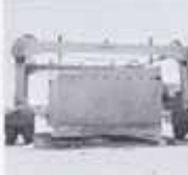
Conventional lifting equipment means concrete boxes are moved slow.
