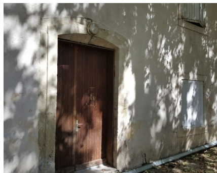
Experimental House Front View
