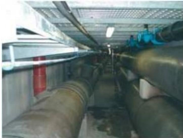
**Figure 6: Utility Gallery, Geneva, Switzerland. The utility gallery is a multifunctional structure which welcomes all types of urban utilities (electricity, water, optical fiber, gas).**
