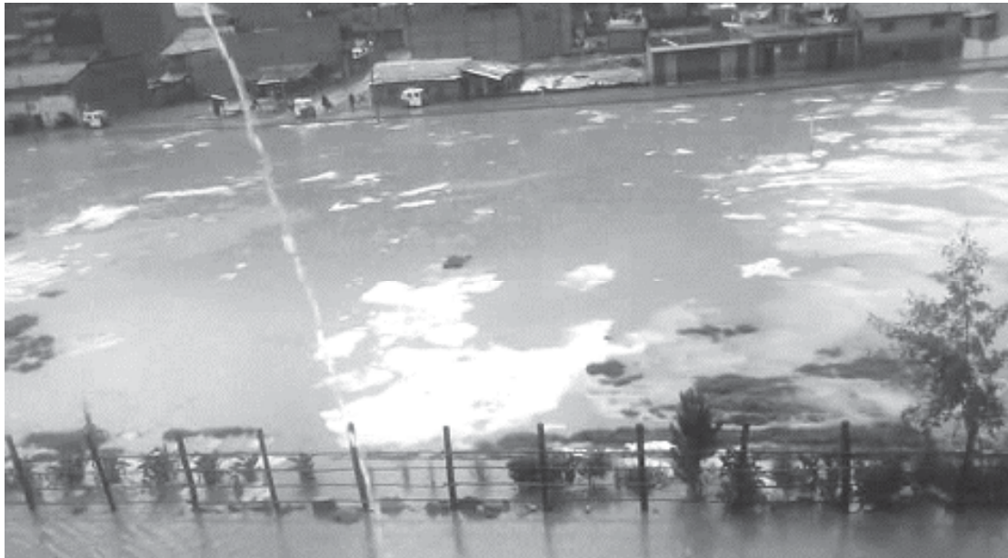
Figure 85: Flood in the recreational area of Purumpampa in 2016.
