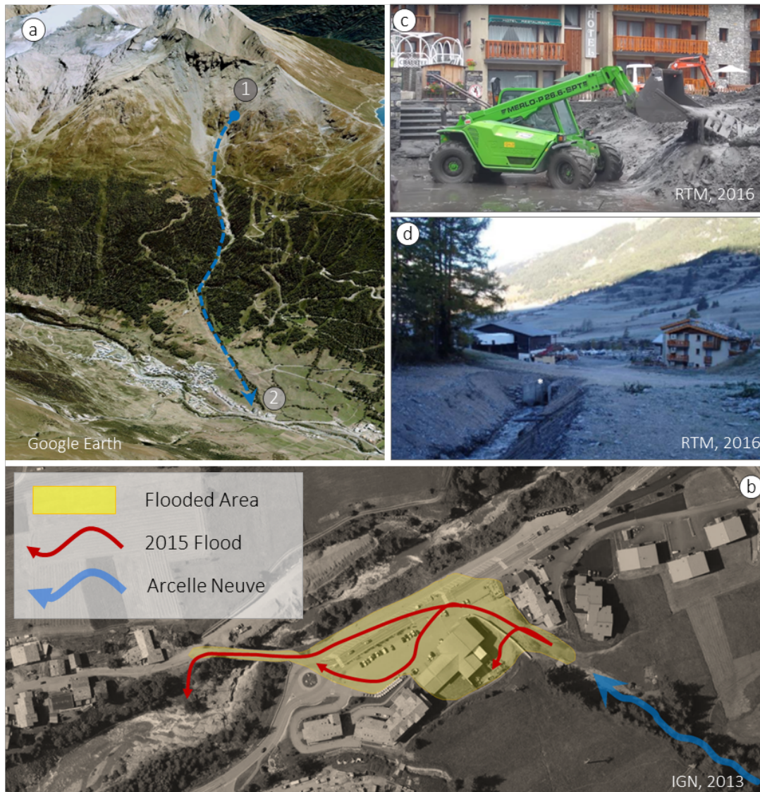
FIGURE 5.2: Overview of the debris flow stages. In (a) is presented the Arcelle Neuve stream, connecting the Lou rock glacier (1) and Lanslevillard (2). In (b) is illustrated the flooded area. In (c) is shown an excavator clearing the area from debris. In (d) is shown a pipe that channels the stream below the town before the confluence.
