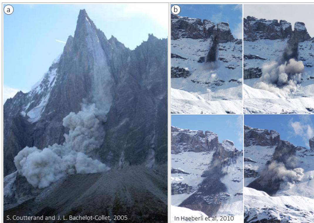
FIGURE 2.9: Rock fall at the Dru (a), and the collapse of a pillar from the Gross Charpf (b), from Haeberli et al. (2010)
