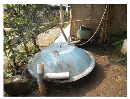
Figure 30 Biogas installation in the farm
