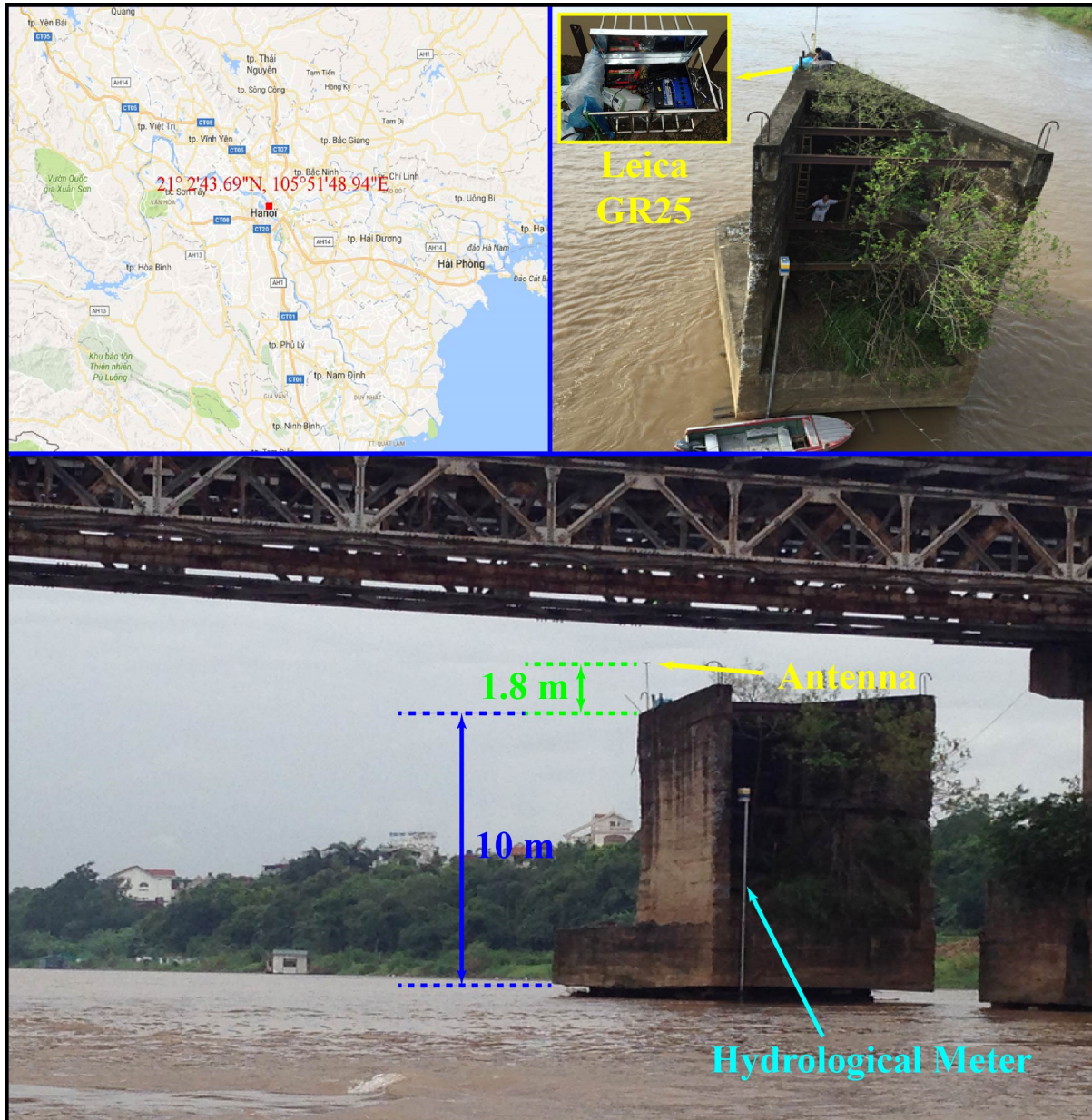
Figure IV.15 – The GNSS receiver with a single antenna installed on the top of the old bridge abutment ( 21^{\circ}2'44.04''N, 105^{\circ}51'48.86''E ) on the Red river in Hanoi, Vietnam from the 27 th July to 12 th August 2016. (Ha, 2018)
