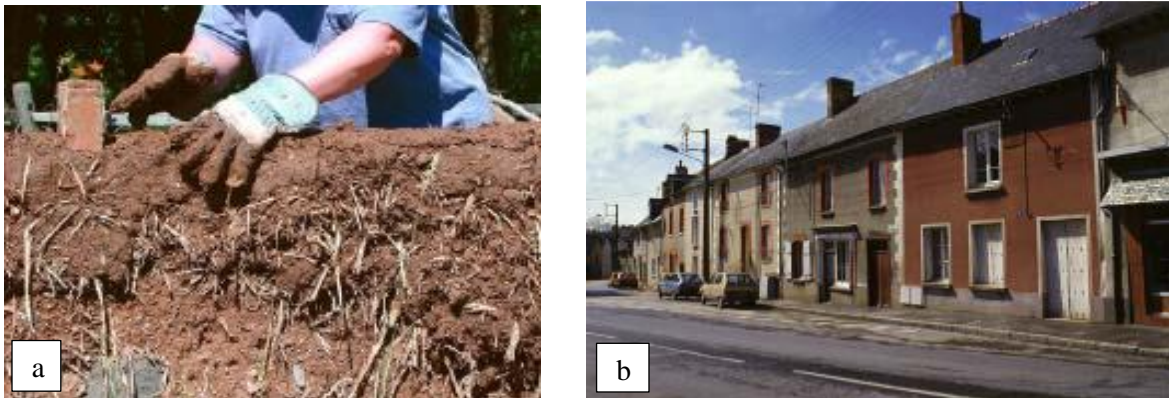
Figure 1.6 (a) a wall under construction with cob (b) a house using cob technique in Ille-et-Vilaine France
