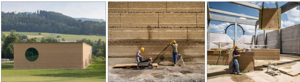
Figure 1.9 Prefabricated rammed earth wall used to build Ricola’s factory in Switzerland
