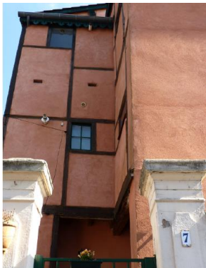
(a) Wattle and daub constructions, Lyon, France
