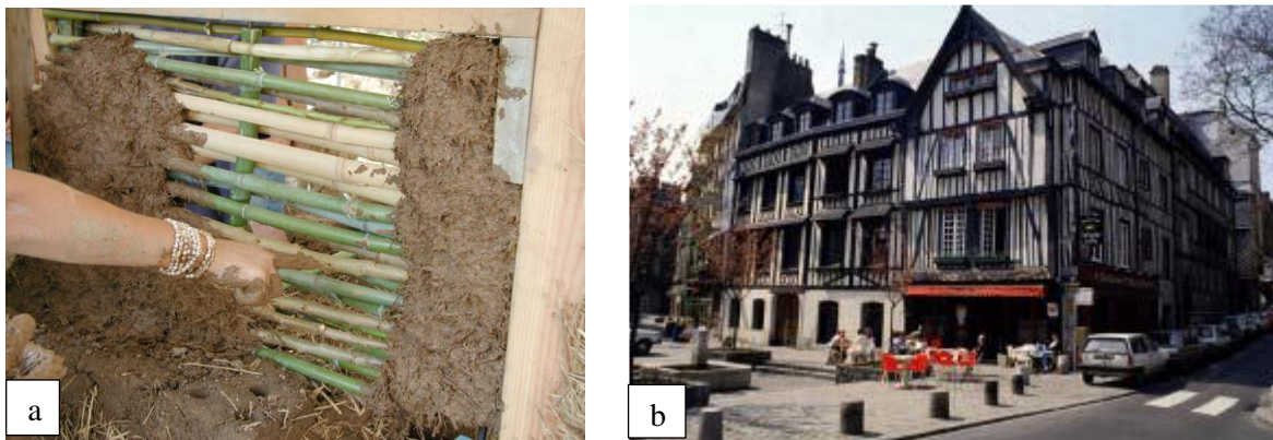
Figure 1.3 (a) construction process using wattle and daub technique (b) house made of wattle and daub in Colmar France
