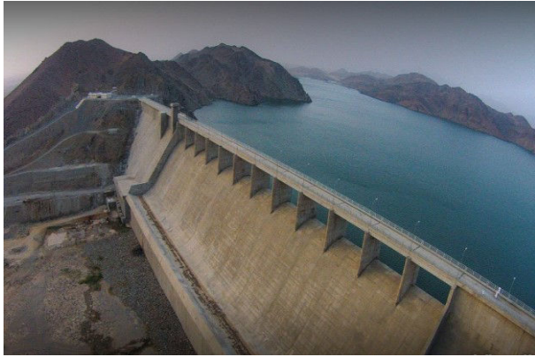
3- Hali dam in Makkah.
