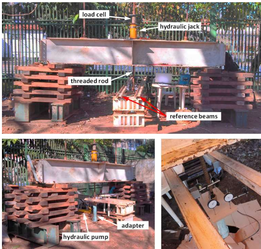
Figure 44. Load test setup.
