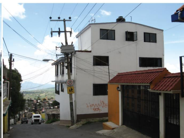
Photo 4.22. C. Zapata, San Pablo Oztotepec, DF [2011]
